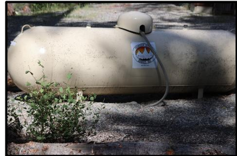
This propane is distanced properly from the home and has an adequate gravel base.
