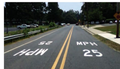
FIGURE 1. EXAMPLE OF SPEED LIMIT ON PAVEMENT
